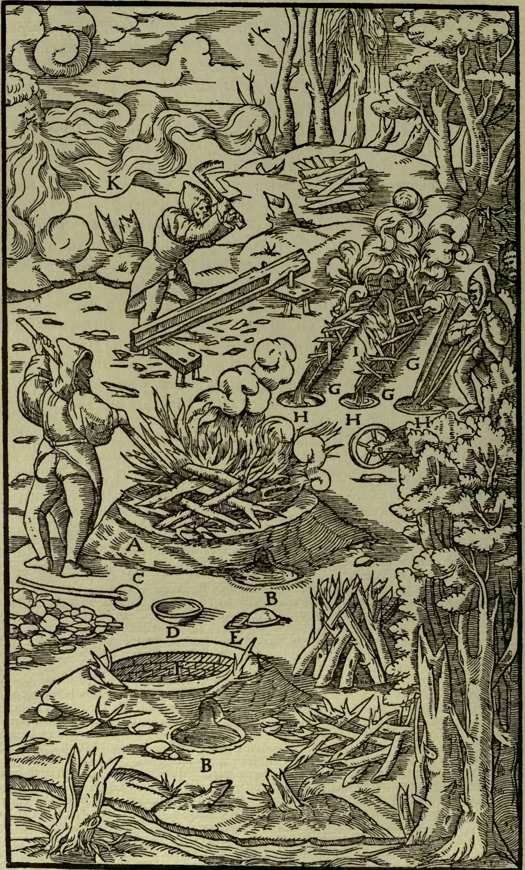
A—PIT ACROSS WHICH WOOD IS PLACED. B—FOREHEARTH. C—LADLE. D—IRON MOULD. E—CAKES. F—EMPTY POT LINED WITH STONES IN LAYERS. G—TROUGHS. H—PITS DUG AT THE FOOT OF THE TROUGHS. I—SMALL WOOD LAID OVER THE TROUGHS. K—WIND.
