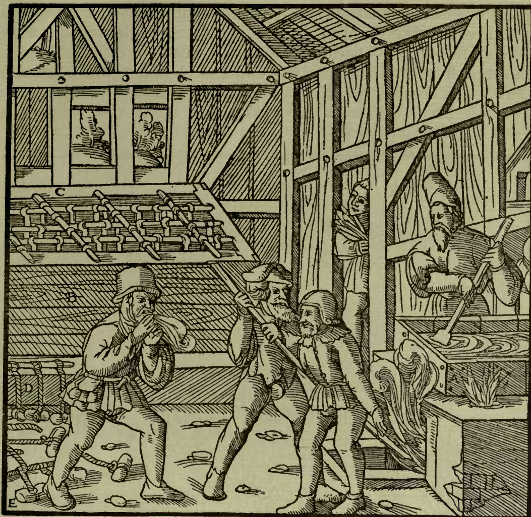
A—CALDRON. B—TANK. C—CROSS-BARS. D—ROPES. E—LITTLE STONES.
