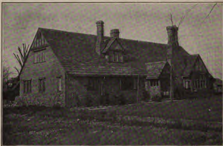
Fig. 89. — By decreasing the exposed length of shingles toward the top a greater apparent expanse is obtained.
