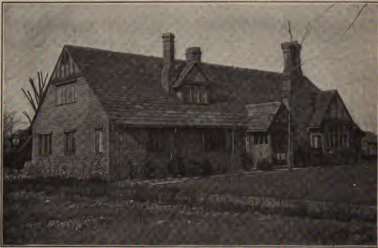
Fig. 89. — By decreasing the exposed length of shingles toward the top a greater apparent expanse is obtained.
