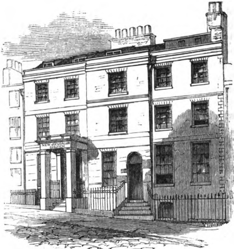
LADY HATTON'S HOUSE, CROSS STREET, HATTON GARDEN.
