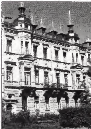
Houses of the brothers Theodore and Bernard, Hornschuchpromenade 3 and 4 (image from The Historical Society Fürth)
