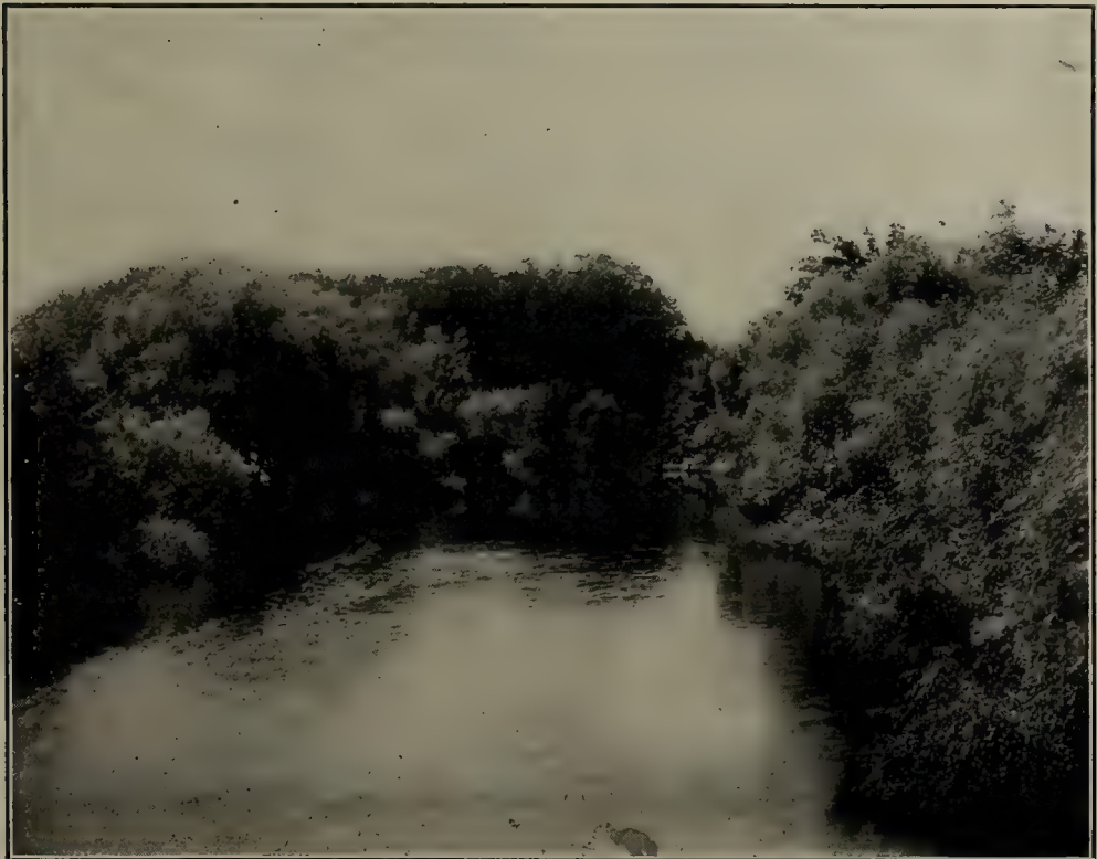
FISH CREEK, OPENING OF WOOD CREEK, which will be a part of the Barge Canal.
