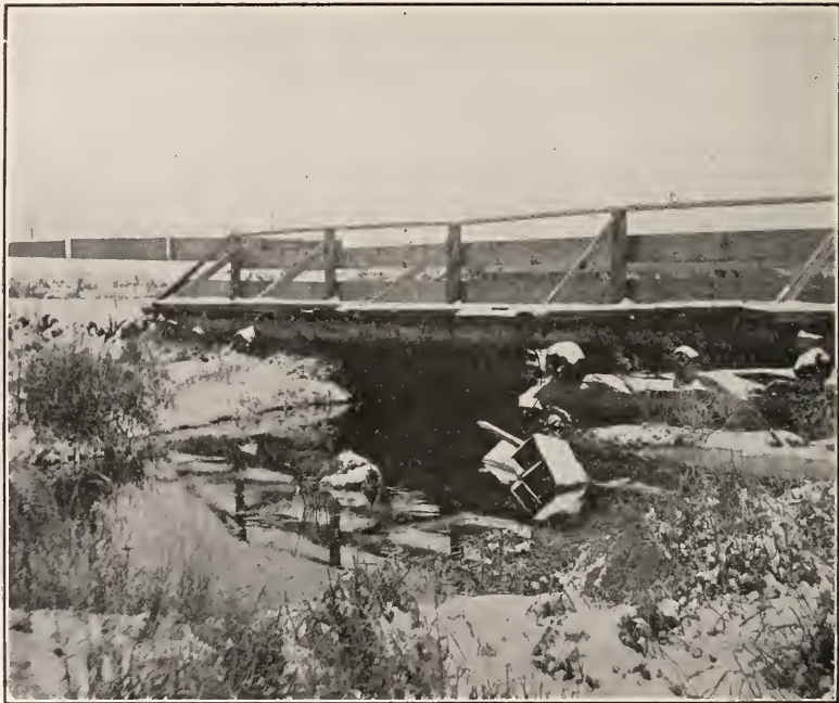
CREEK WHERE SEWAGE EMPTIES.
