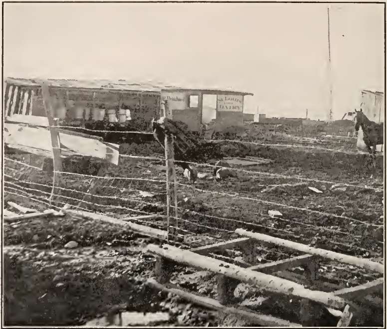
MILK HOUSE, showing the close proximity of a privy which was open to flies. The privy is the shed just behind the horse. The horse is standing in the drain from milk house, which was being used as a wallowing place for pigs.
