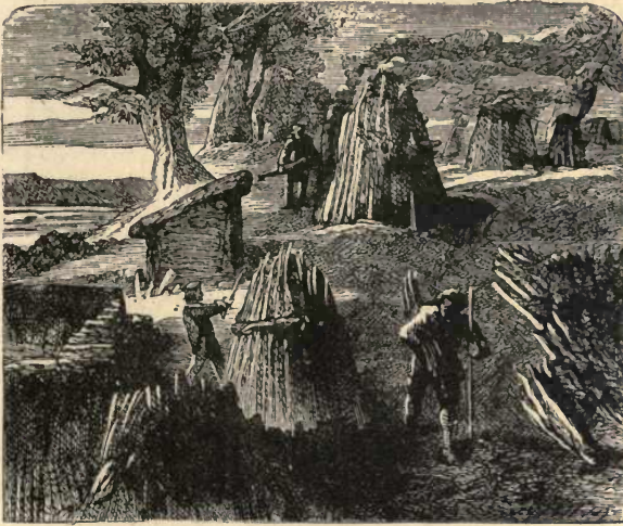
Fig. 368.—Wood piles of charcoal burners.
