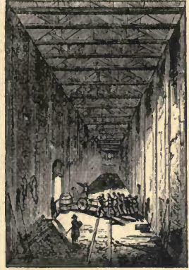
Fig. 390.—Plate-glass casting—bringing out the pot.
