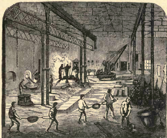
Fig. 403.—General foundry, Woolwich Arsenal.
