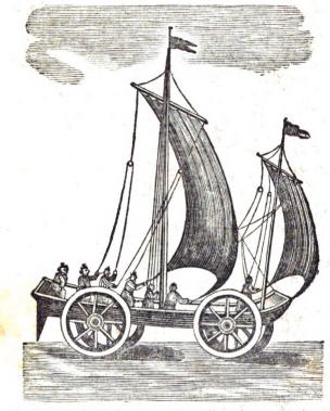
The body of it being somewhat like a boat, moving upon four wheels of an equal bigness, with two sails like those in a ship; there being some contrivance to turn and steer it, by moving a rudder which is placed beyond the two hindmost wheels; and for the stopping of it, this must be done, either by letting down the sail, or turning it from the wind.
