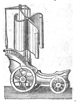
In which the sails are so contrived, that the wind from any coast will have a force upon them to turn them about; and the motion of these sails must needs turn the wheels, and consequently carry on the chariot itself to any place (though fully against the wind) whither it shall be directed.
